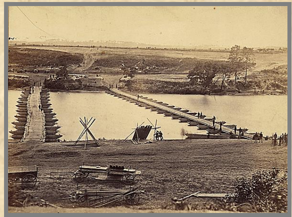
Pontoon Bridge on the Rappahannock River May 1863
