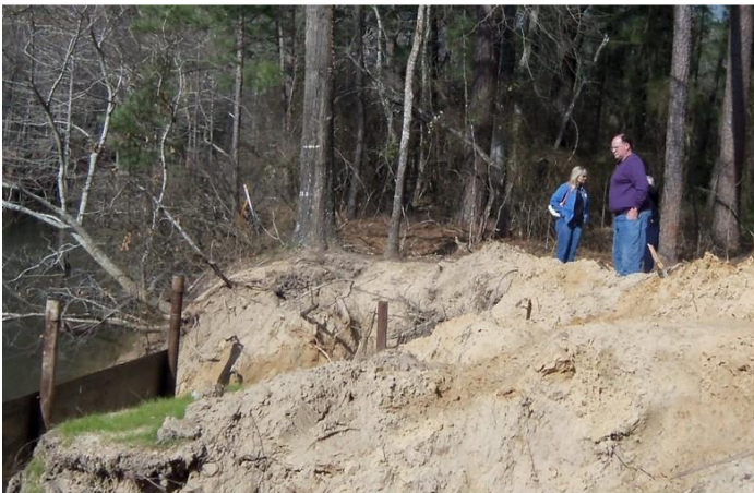
Robbin Hedrick David Routh Recently installed steel embankment stabilizing wall
